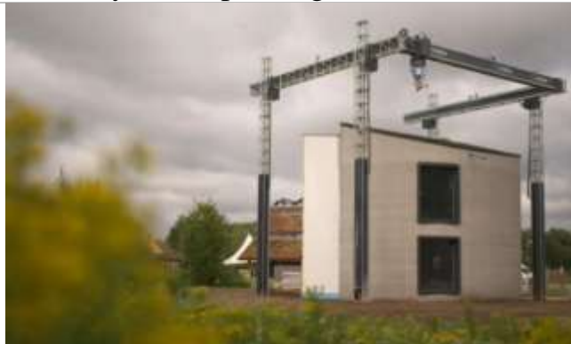
Fig. 1. The COBOD BOD2 printer. Printing is performed using a cementitious mixture.
